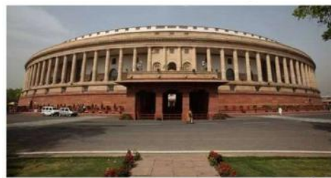
External colonnade façade at the Rashtrapati Bhavan
